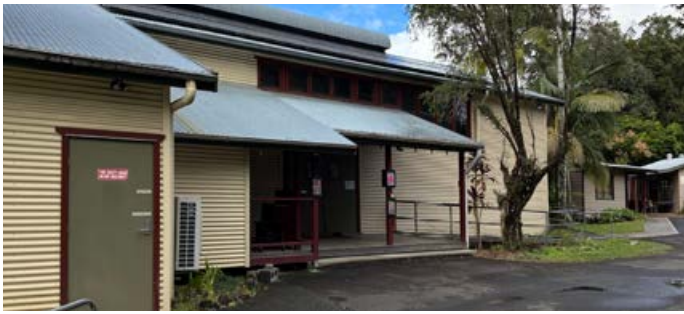
The Drill Hall
