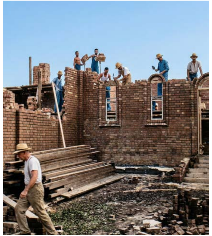
Builders at work at St Kevins Catholic Church
