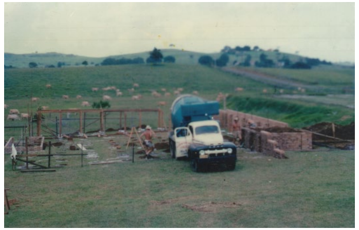
Early construction work at the club Photo from the archive of Jan Hulbert
