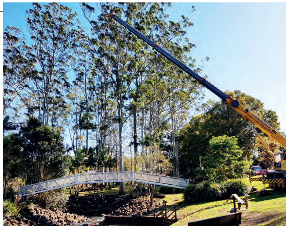
The new bridge being lowered by crane Photo Lynn Smith
