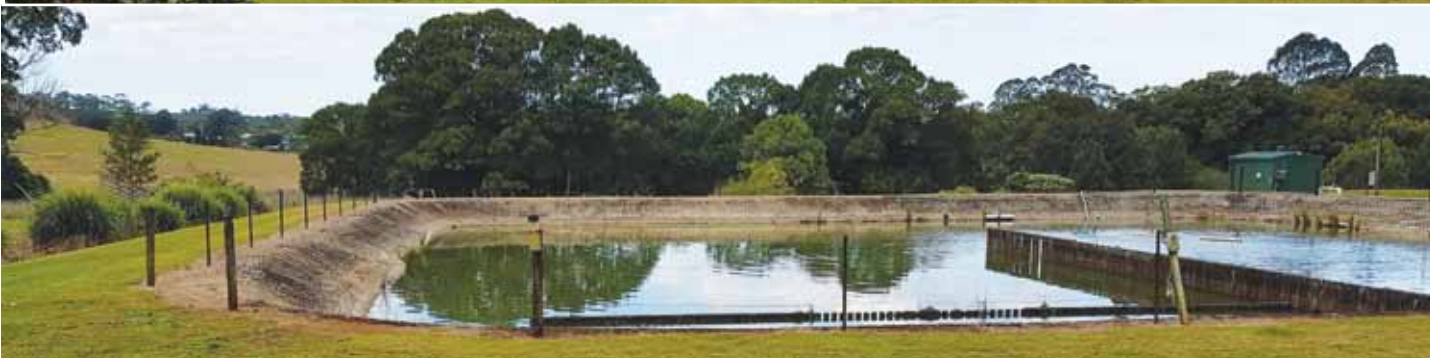
Top, the solar array powering operations. Below: the settling ponds at the Bangalow STP.
