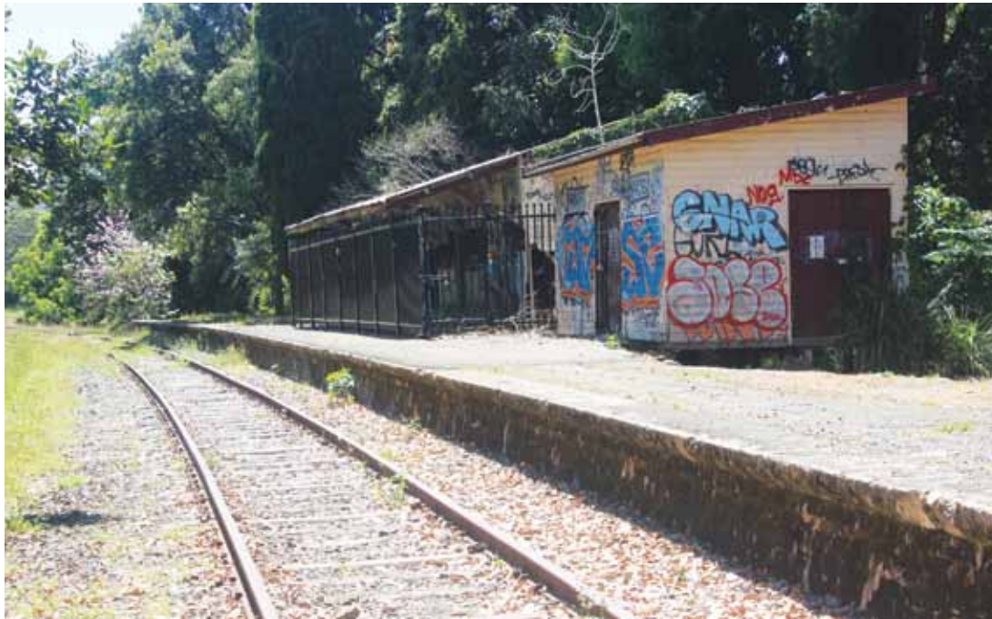
The disused Bangalow Railway Station Photo: Jim Hearn
