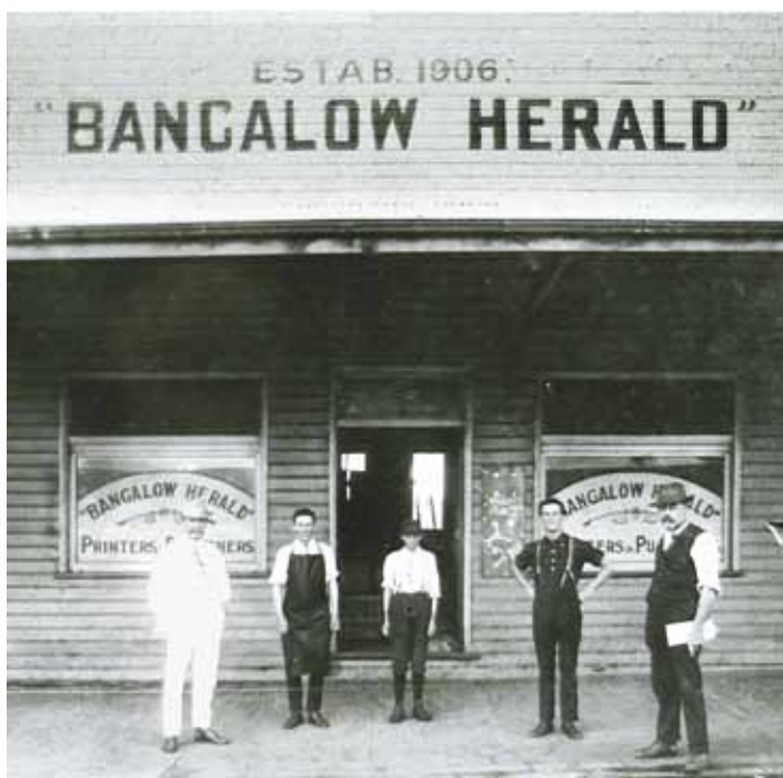
New premises in Byron Street 1908-1920.
