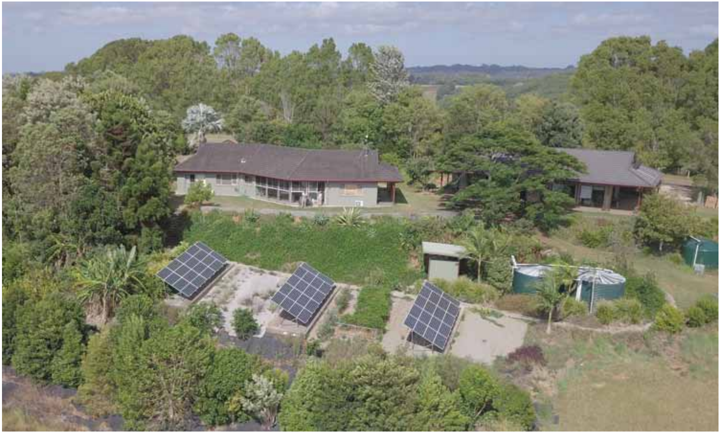
Left: Edible plants grow amongst the solar panels. Photo: Christobel Munson Above: The 54 solar panels provide power for the house and EV. Photo: Al Percival
