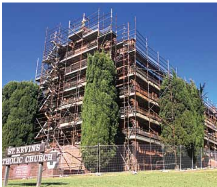
In need of repair: St Kevin's brickwork has a mortar makeover. Photo: Murray Hand
