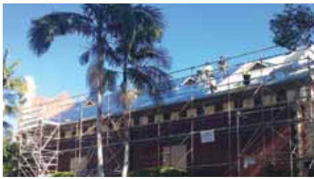
Raising the new (well-insulated) roof on the historic A&I Hall. Photo: Murray Hand
