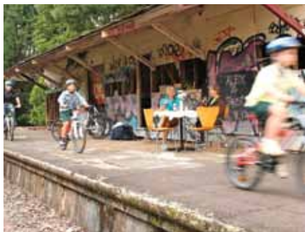
Bangalow station could get an upgrade as part of the Rail Trail project.
