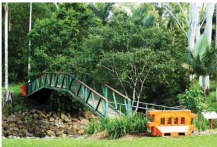
Demolish or replace? What to do with the old bridge is a big question.
